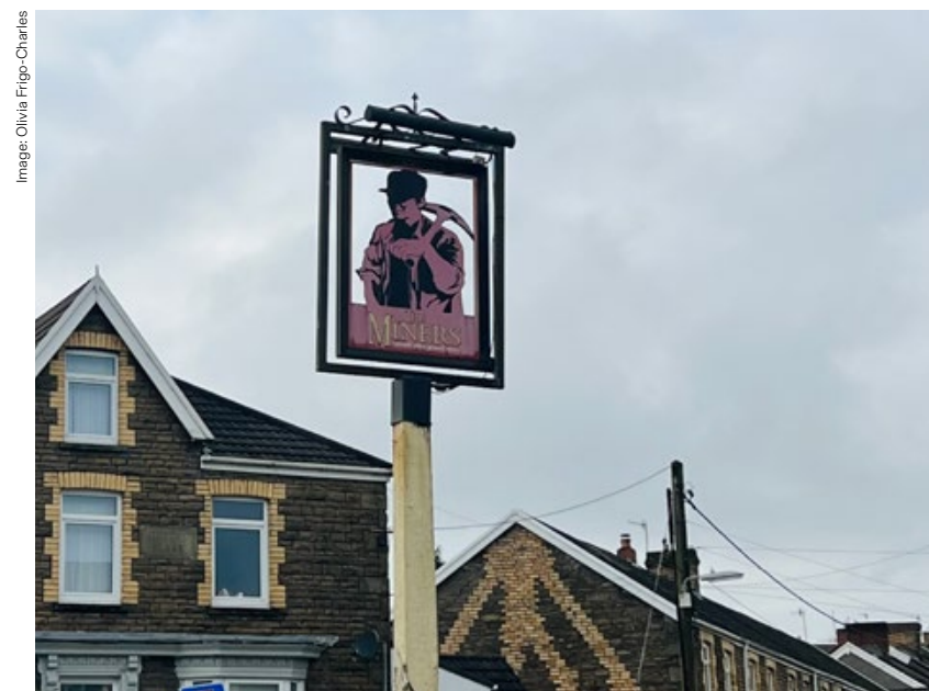
Figure 2: Former 'Miners' Pub' which was recently converted into a grocery shop and flats.
